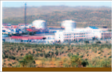
Tazhong Oilfield, China's largest desert oilfield, has 61.3 million tons of proven oil in place and 20.36 million tons of recoverable reserves.
